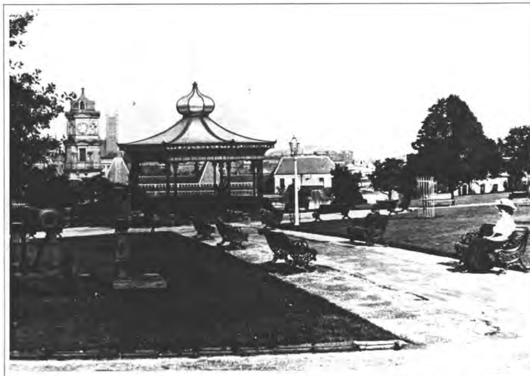
Figure 16 Albert Park bandstand shortly after completion, showing the onion dome, painted floral frieze and trellis cornice, ATL
