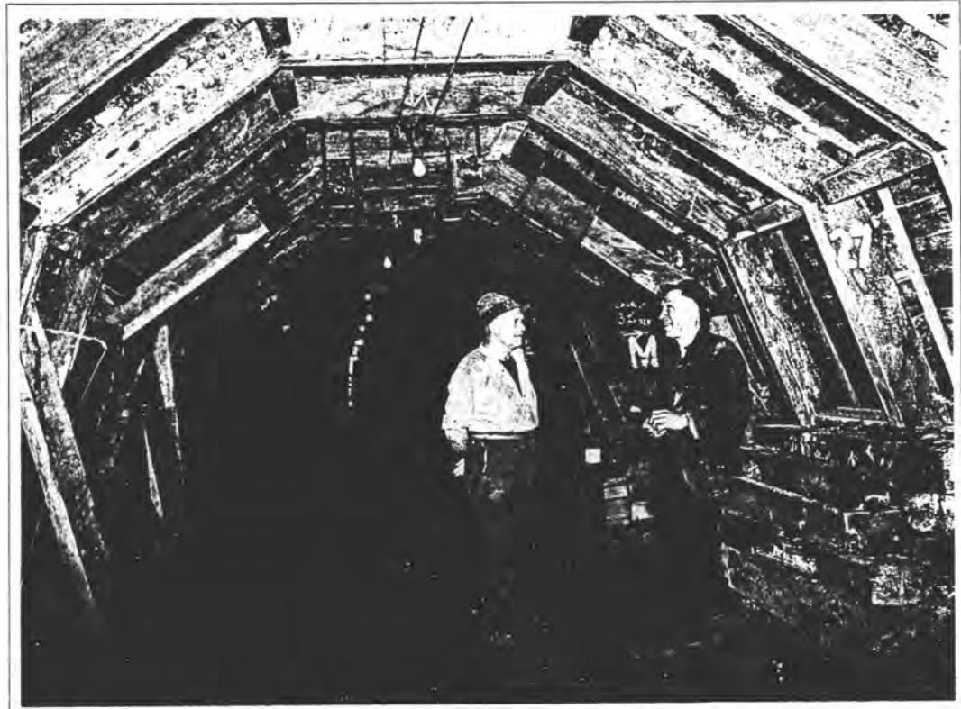
Figure 20 Interior view of a main shaft in the Albert park air raid tunnels, AIM C30109
