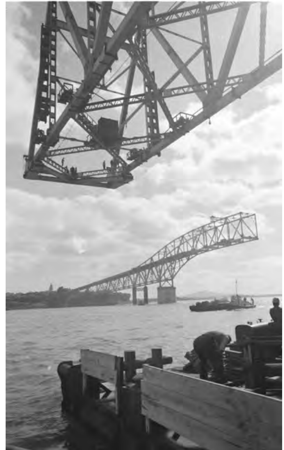
Construction of the Auckland Harbour Bridge (c.1959), Les Downey – Auckland Libraries Heritage Collections 314-A16414.
