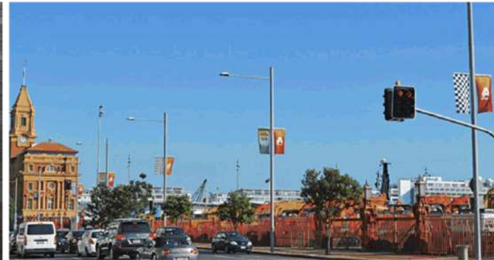
Smart poles for street and intersection lighting
