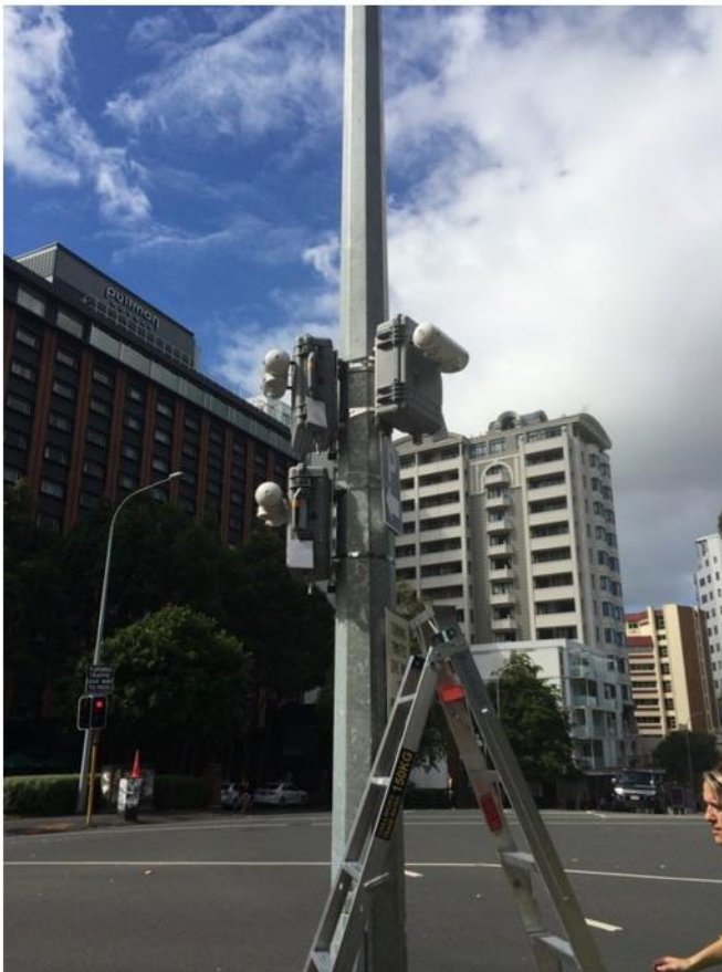
Figure 2-1: Three SpaRTANZ air samplers installed on Princes Street, Auckland.
