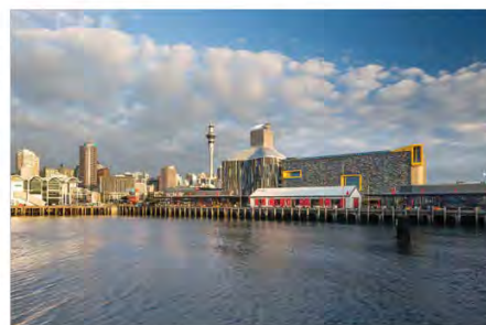
Top Left: North Wharf from new breakwater Bottom Left: North Wharf from end of Halsey Wharf breakwater
