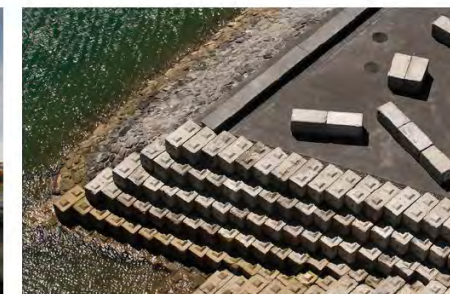
Top Right: Precast steps on access to water Silo Park edge Bottom Right: Silo Park western edge
