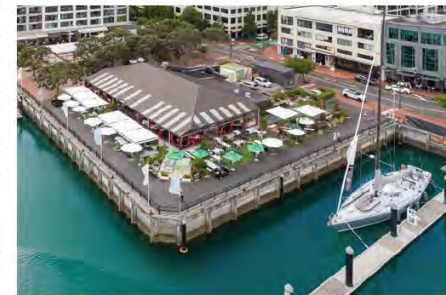
Left: Inner Viaduct adjacent to old Headquarters site
